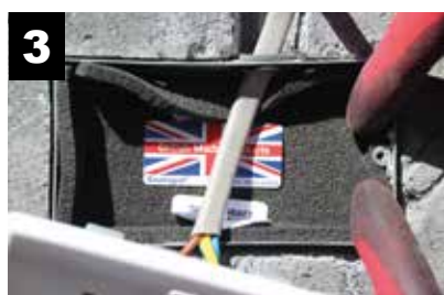
Insert the gasket and press firmly to attach to the box.
