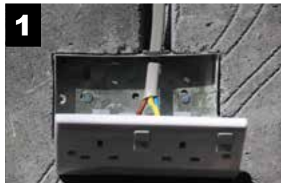
Insert the metal box into the wall.
