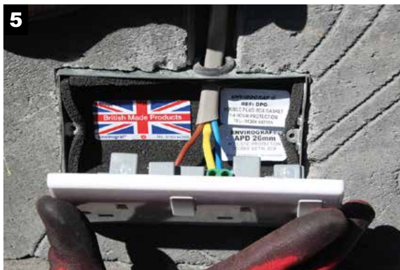
Job done. You now have fully fire and acoustic protected metal box.
