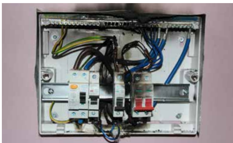
Plastic Consumer unit extinguished by EnviroBurst
