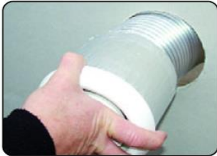
STEP 4: fit the Firoblok sleeve over the vent and fit to the ducting
