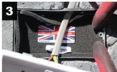
3 Insert the gasket and press firmly to attach to the box.
