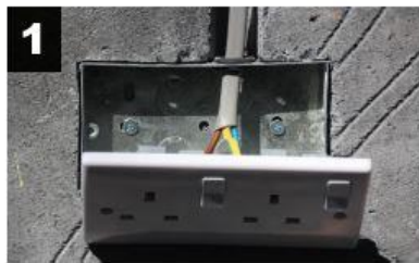
1 Insert the metal box into the wall.
