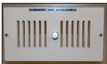
Vent in open position
